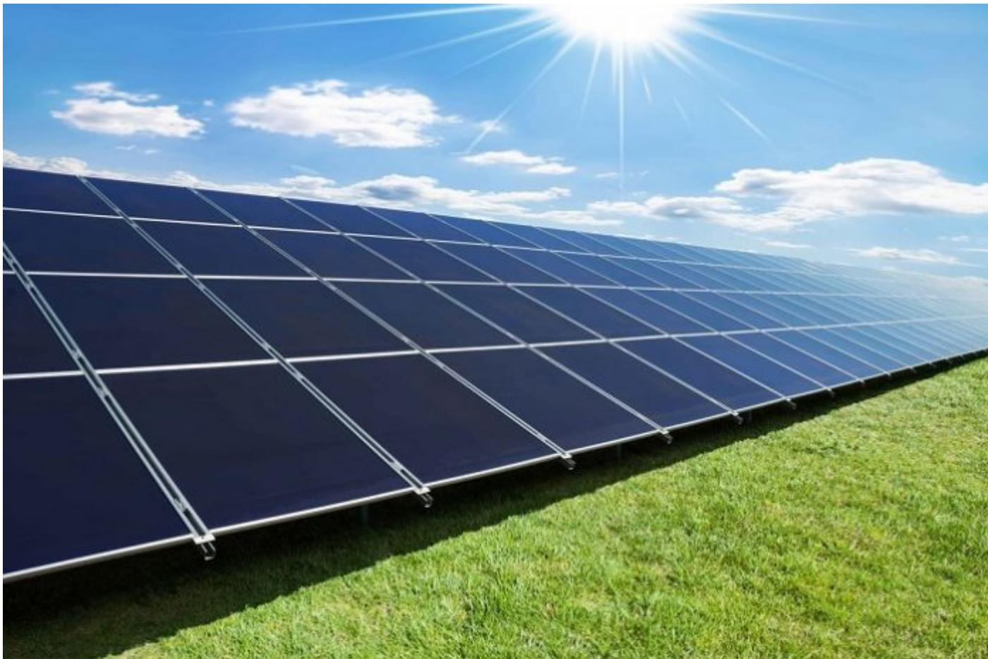
Solar panel (also known as "PV panel") is a collection of solar cells that are made to absorb light as a source of energy and convert it to electricity that can be used in a range of applications including commercial and residential applications.
